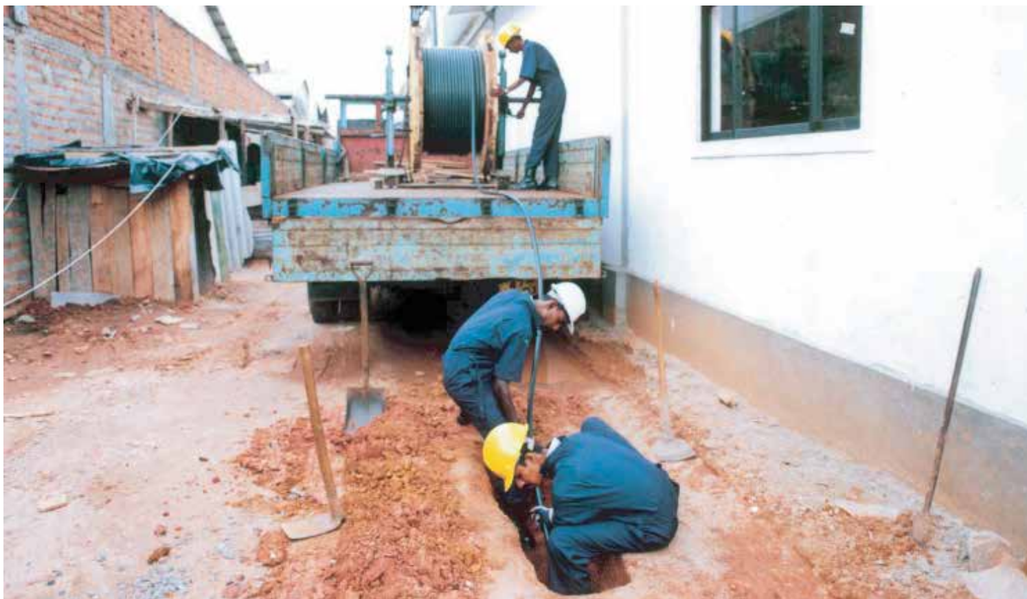
Installing Power-X Cable
