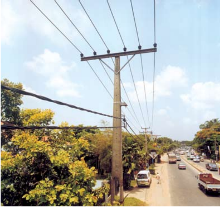
Two Aerial Bundled Cables running parallel to each other. Example of easy augmentation
