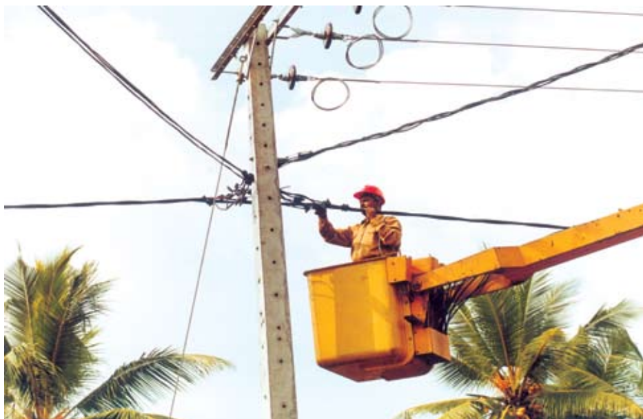
Technician inspecting an installed ABC line
